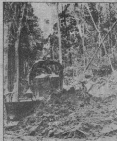
ROADS To remove short lengths, or "snigging" of logs to motor transport, gravel surfaced roads are driven as close as practicable to felling sites. Powerful bulldozers quickly cut a swathe for roadway through timber.
